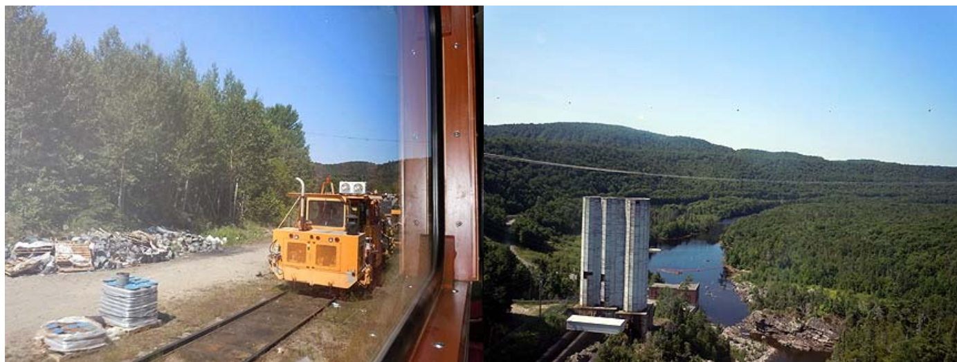
Evidence of ongoing work on the tracks
