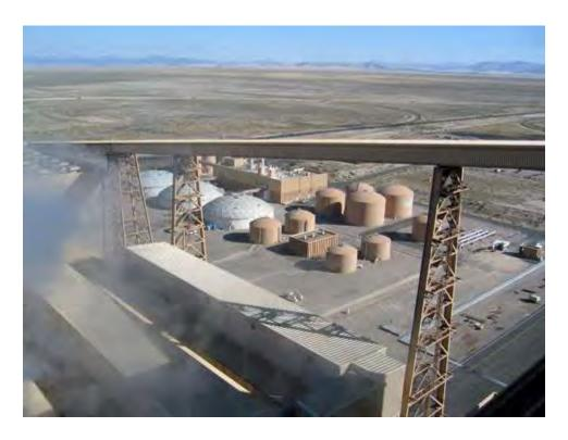
This is the coal conveyer. Two 100 car trains per day bring coal to the plant. It is crushed to the consistency of baby powder, and blown into the boilers.
