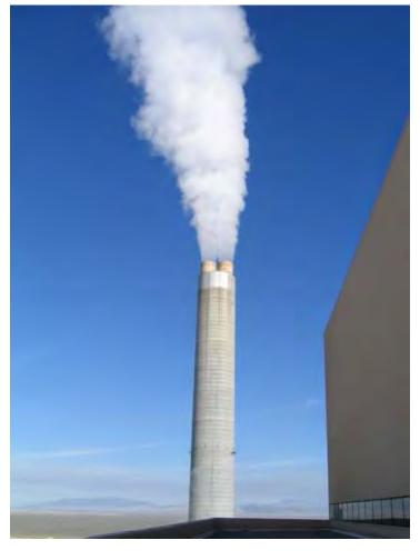
The 700 foot chimney and related scrubbers and baggers remove over 99% of the ash, and over 95% of the sulfur dioxide. The project burns 10 tons of coal per minute! That's over 4.7 million tons per year.
